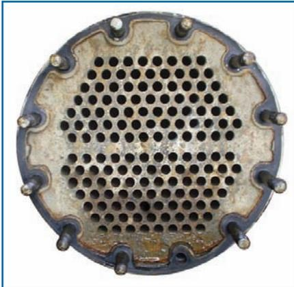
**Picture 1: A clean condenser, treated with BacComber. It remains clean year after year, saving tremendous energy and enhancing condenser life**
