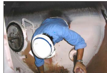
Boiler Drum Inspection
