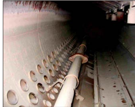
4th Inspection March 05
