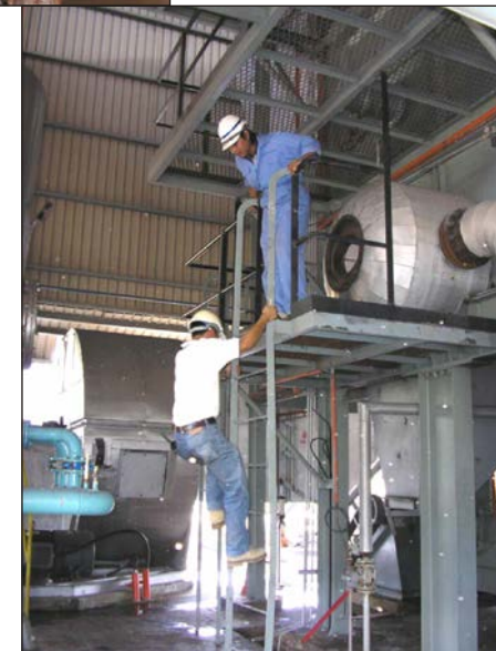
Boiler Drum Inspection
