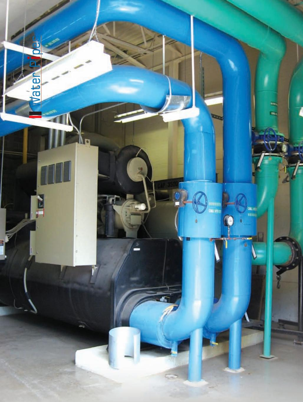
In Pharma companies a pin hole in the chilled water pipeline would mean partial closure of the manufacturing facility and loss in production. Quite often a sample taken from chilled water pipeline is reddish in colour due to rusting. BacComber Treatment has
